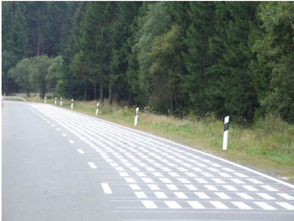
Picture 1 Test field in the Harz Mountains, Germany
